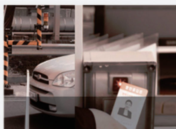
Access security system
